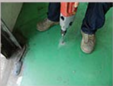
STEP 4 Drill holes 3" deep (drill bit included) -Note- Make sure holes are clean before insertion
