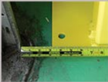
STEP 2 Measure 3" from door rail. Be sure ballard is 1 1/2" covering door rail protection
