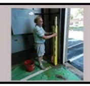
Pour concrete around tube and insert upright tube into sleeve insert while concrete is wet, properly level tube and remove upright tube. allow 2-3 days to cure
