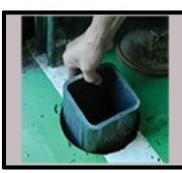
**STEP 5**Insert steel tubing sleeve
