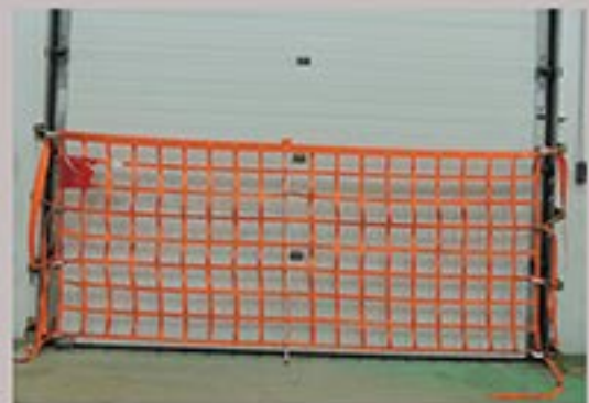
Loading Dock Safety Net Properly Installed
