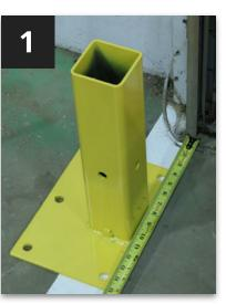
1. Clean the area. Measure 3" from door rail and place post base with at least 1.5" coverage of the door rail. Mark the holes with the enclosed marker.
