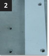
2. Drill holes 3" deep with included drill bit. Note: Make sure to keep inside of holes clean of debris.
