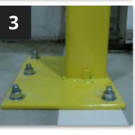
3. Place base over holes and insert anchor bolts with washer and nut.
