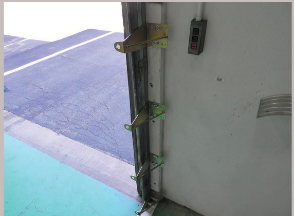
Properly Mounted Brackets
