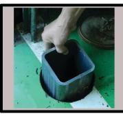
**STEP 5**Insert steel tubing sleeve
