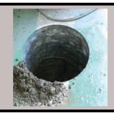
**STEP 4**Remove insert and clean hole of debris
